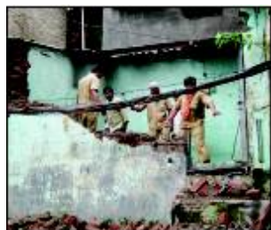
Demolition being carried out on Tansa main in Bhandup in August
