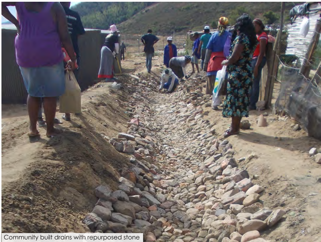
Community built drains with repurposed stone
