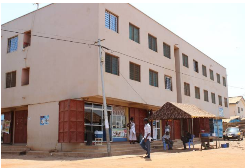
Amui Dzor Building, Ashaiman
